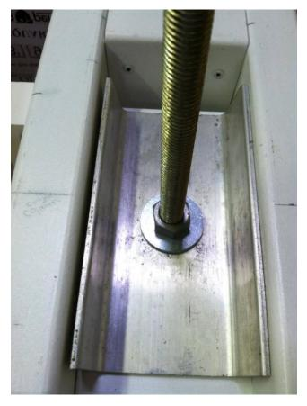
Leave bolt loosely tightened until false beam is installed.
