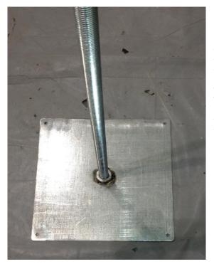
Insert threaded rod into steel bottom plate with nut and washer on each side of the plate. Do this for each of the four plates
